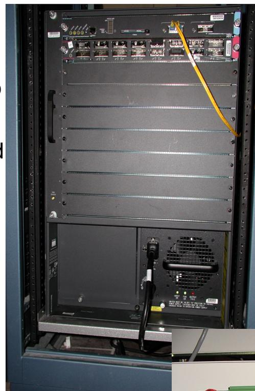
Prototype Control System network core switch.
