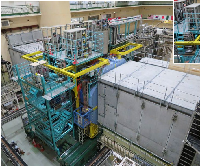
Concrete shield disassembly work
