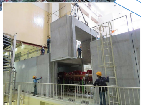
Concrete shield disassembly work
