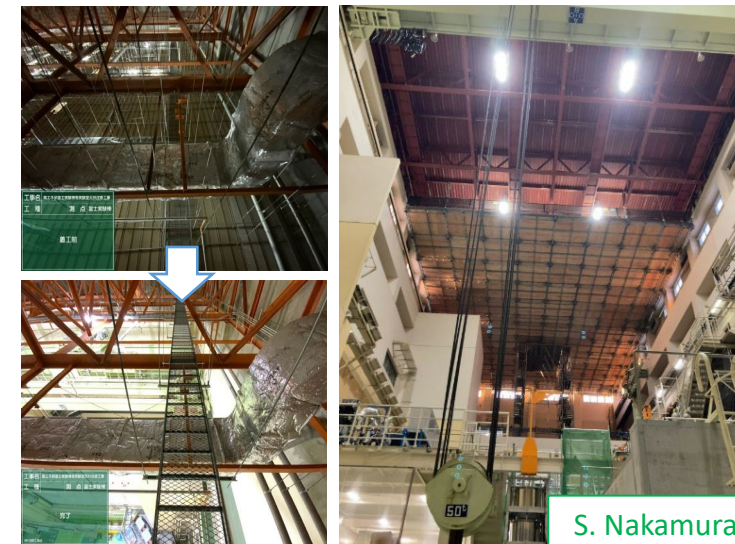
Ceiling aseismic reinforcing work
