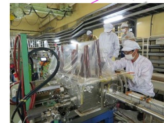
Beam pipe realignment at LER inj. point
