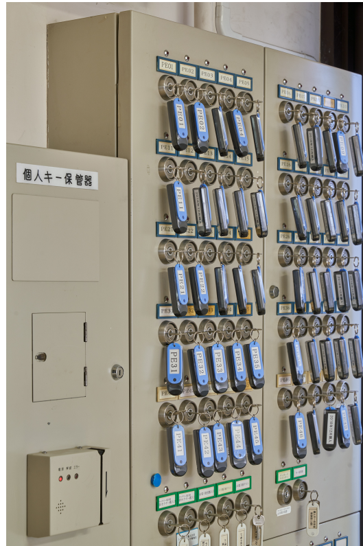
Figure 12.101: Personal keys used for entrance to the linac tunnel and the key bank.
