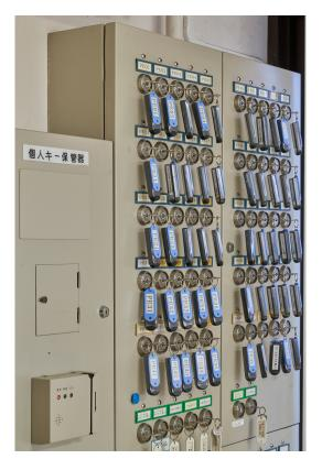
Figure 11.101: Personal keys used for entrance to the linac tunnel and the key bank.
