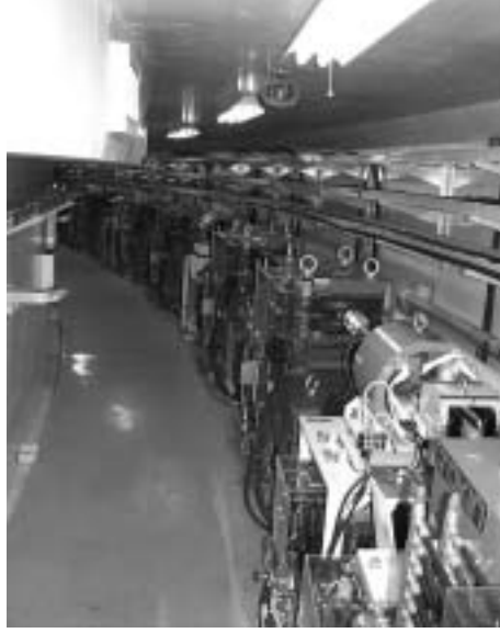
Fig. 3. Typical view from upstream at Arc-1.
