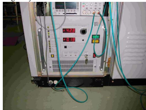
Figure 10: Photograph of the inverter power supply. The size is 449mm(H)x 480mm(W)x 630mm(D).
