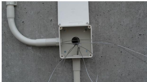
Figure 4: Penetration hole viewed from the east-side wall surface of the linac building for passing thermocouples. The signals of the thermocouples are sent from the outside to a data logger unit installed in the inside.
