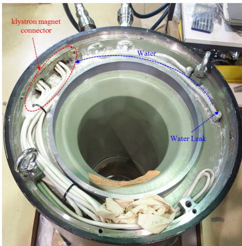
Figure 6: Klystron magnet water leak point.
