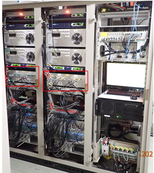
Figure 1: Power supply system for pulsed magnets. In addition to pulsed power supply, control system, interlock system, DC power supplies for charging capacitors of the pulsed power supplies are shown. Each unit feeds 8 ch pulsed magnets. Bipolar power supplies for pulsed steering magnets are indicated by red rectangles.
