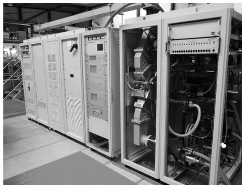
Figure 3: 30 kW IOT based transmitter
