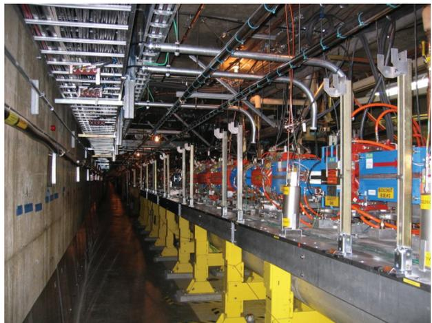
Figure 4: Sector 20 with the new FACET magnets installed.
