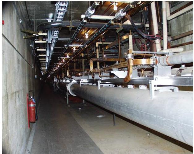
Figure 3: Sector 20 before the accelerator systems were removed to make way for FACET. The linac is visible above the much larger alignment light pipe.
