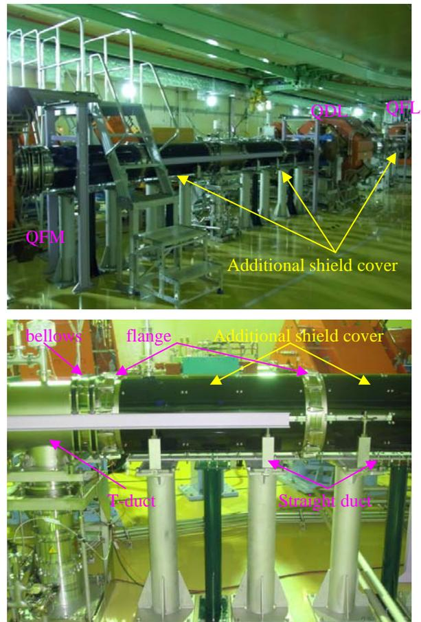
Figure 5: Photo of the RCS ring duct wrapped with the additional shield covers.
