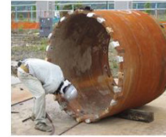
Casing Bit for Excavation
