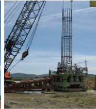
Reinforcing Rod of Pile
