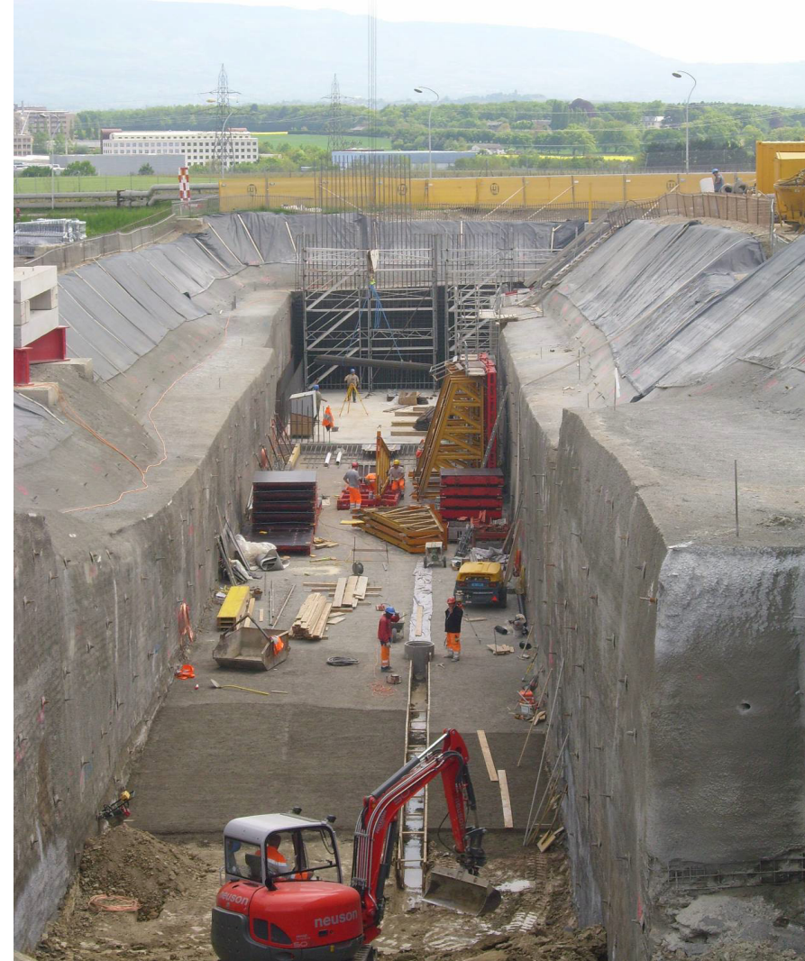
Excavation work, April 2009
