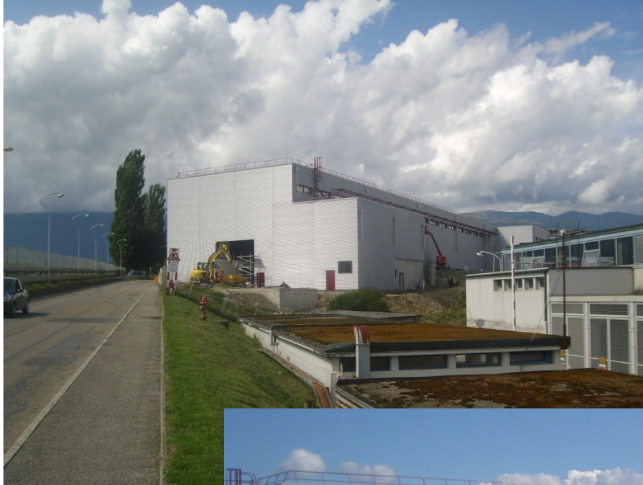
Surface building, August 2010
