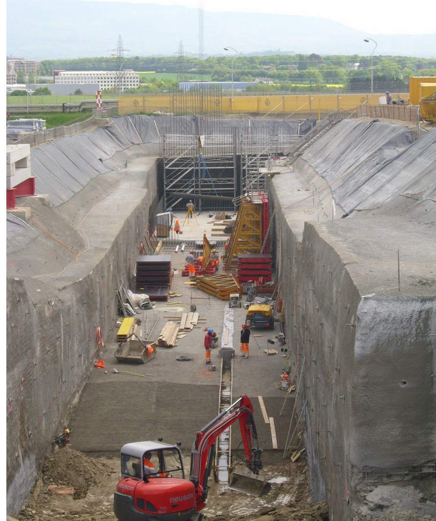
Excavation work, April 2009
