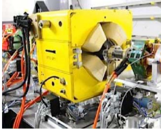
Figure 6: Replacement QF1FF magnet installed at ATF2. Quadrupole magnet previously used as an arc quad in the LER ring at PEP-II, SLAC.
