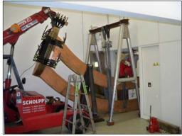
Bringing-in procedure of the 90° gantry dipole spare coils into the gantry hall.
