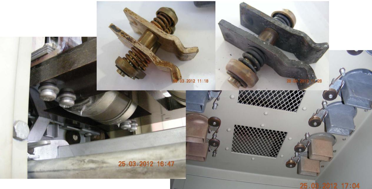
SUB 22 400V ac Bus-Coupler – 3 days lost. No spares! Redundancy is arranged by the operation of the bus coupler. Unfortunately the unit had not been serviced for some time as it was scheduled to be replaced. Problem due to weak springs on the fuse carrier receptacle.
