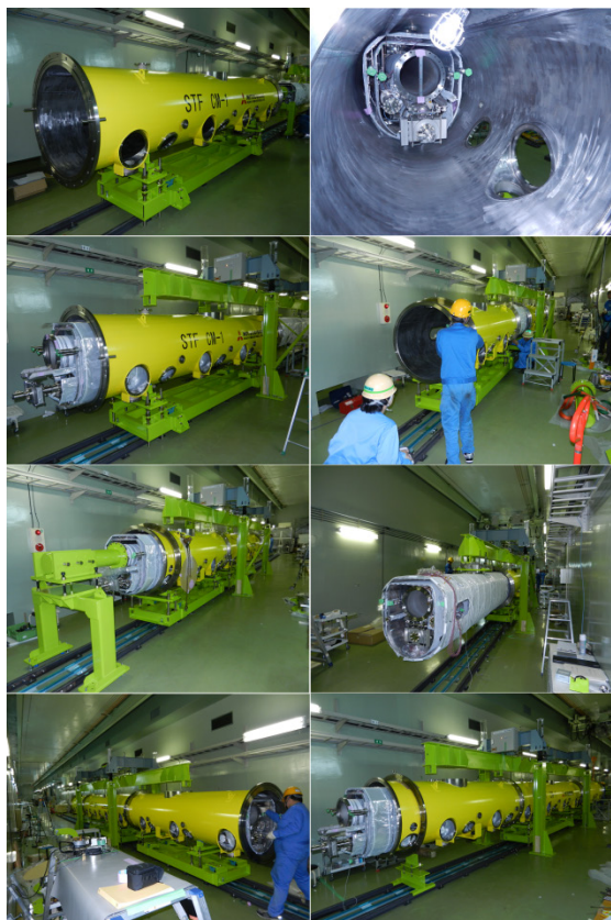
Figure 8: Insertion of 8 stringed cavities into the cryostat in the STF tunnel : MHI#14~MHI#22 without MHI#16.
