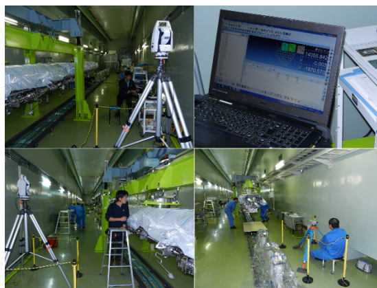
Figure 7: Alignment of the cavities hanging under the Helium return pipe (GRP).
