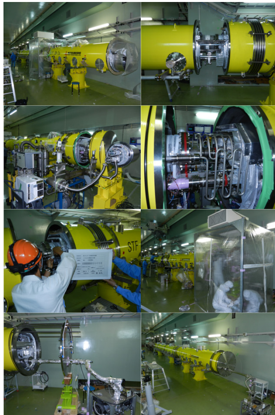
Figure 10: Connection between CM1 and CM2a cryomodules.
