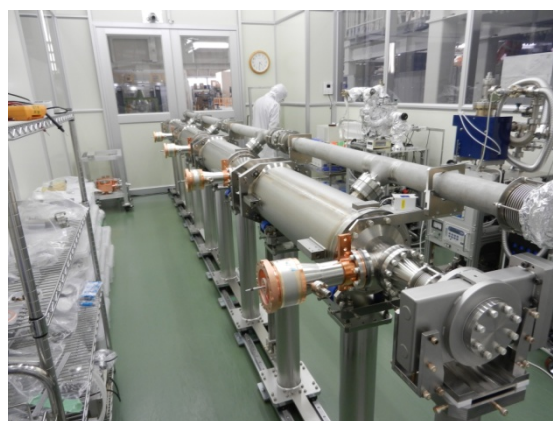
Figure 4: String assembly of 4 cavities : MHI#19 ~ MHI#22.
