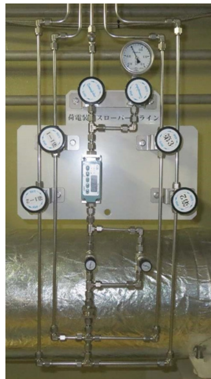
Figure 2: Photograph of the centralized gas flow control unit for the slow purging system.
