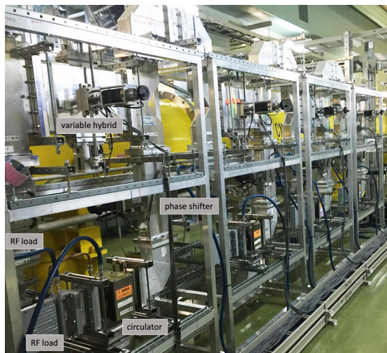
Figure 9: Close picture of the RF power distribution for 4 LPDS system. The one unit consists of variable hybrid, phase shifter, circulator, and RF loads. Behind this LPDS, there is cavity power coupler which is connected to the #2 port of the circulator. RF power flow is from the left to the right.
