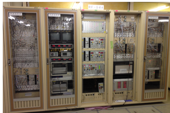
Figure 4: Old LLRF control system, which was used in KEBK operation, continues in use for SuperKEKB.
