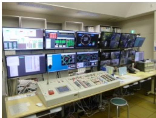
Figure 5: The safety system console.
