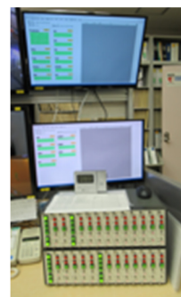
Figure 7: The access control system console.
