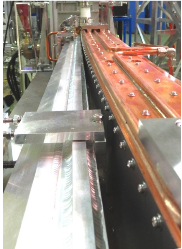
Figure 4: New Al-alloy stored beam duct installed next to the S2 magnet. Cooling water channels are welded on top and bottom of the beam duct to remove the SR heat load along the tapered wall on the S2 magnet side.
