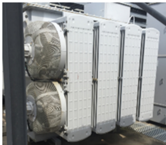
Figure 2: MR-RF transformer-rectifier unit.
