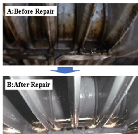
Figure 3: Repair of the radiator. A: before repair, B: after repair.
