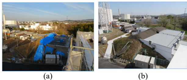
Figure 7: (a) Under repair. (b) Complete repair.
