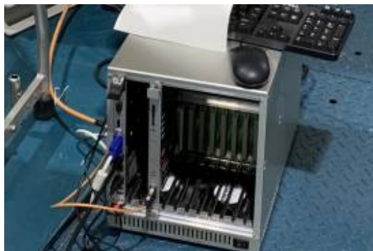
Figure 5: MTC with newly installed VME CPU.
