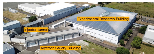
Figure 1: NewSUBARU synchrotron light facility.
