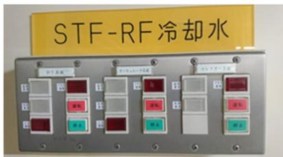
Figure 2: Cooling water operation switch.
