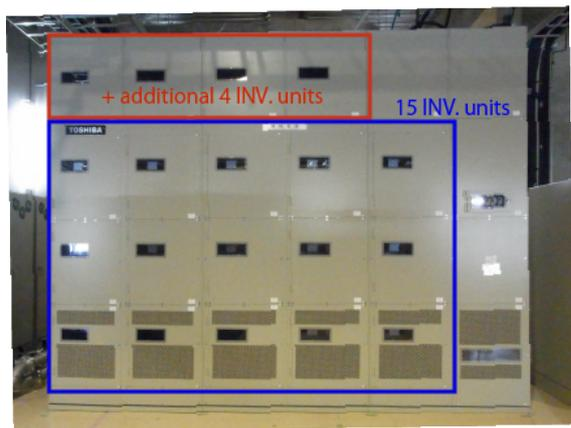
Figure 1: Anode power supply with 19 inverter units.
