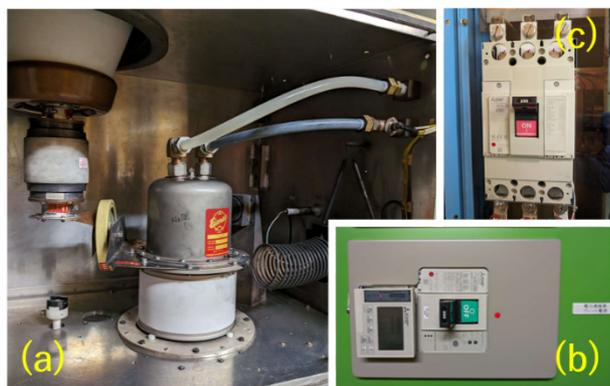
Figure 6: Replaced devices for AVF. (a) Vacuum tube, (b) ELCB, (c) MCCB.
