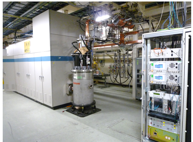
Figure 1: Layout of RF source and RF monitor rack.
