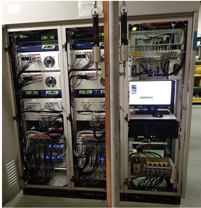
Figure 11.41: A photo of the standard unit for 4 quad and 4 steering magnets.
