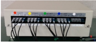
Figure5: Photograph of the control unit.
