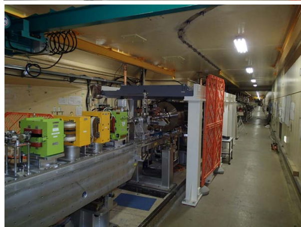
Figure 1: The radiation shield at the unit#1-5. Before and after the shield installation (Top and bottom).
