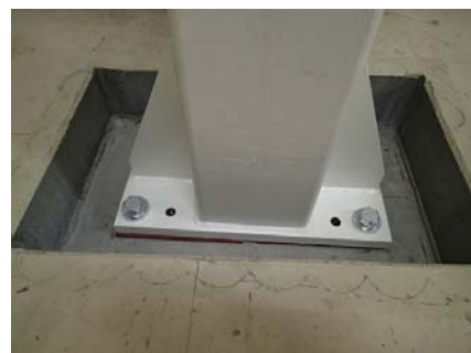
Figure 4: Column base plate
