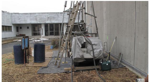
Figure 2: Preparation of boring devices and a boring point in the 17.6 m north from the entrance of the injector linac building.
