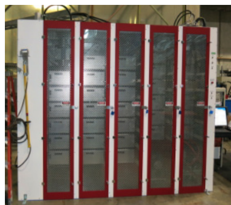
Figure 7: Photograph of the P2 Marx modulator.
