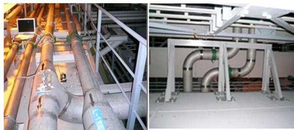
Figure 13: Sensors on the L1 pipe(left). Looking up L1 pipes on the support from maintenance path (right).
