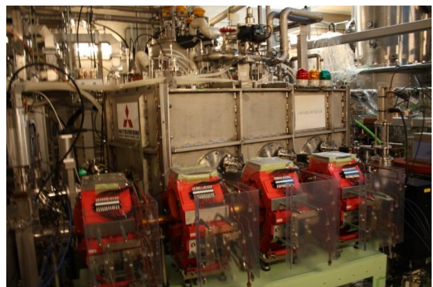
Figure 2: Injector cryomodule installed in the beam line.
