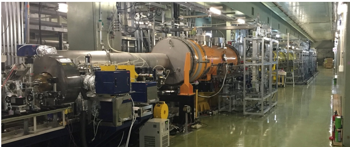
Figure 1: Tunnel view of the STF accelerator. The RF power distribution system is installed in the right side of capture cryomodule, CM-1 and CM-2a. Vector sum field control was demonstrated for 8 cavities combined.
