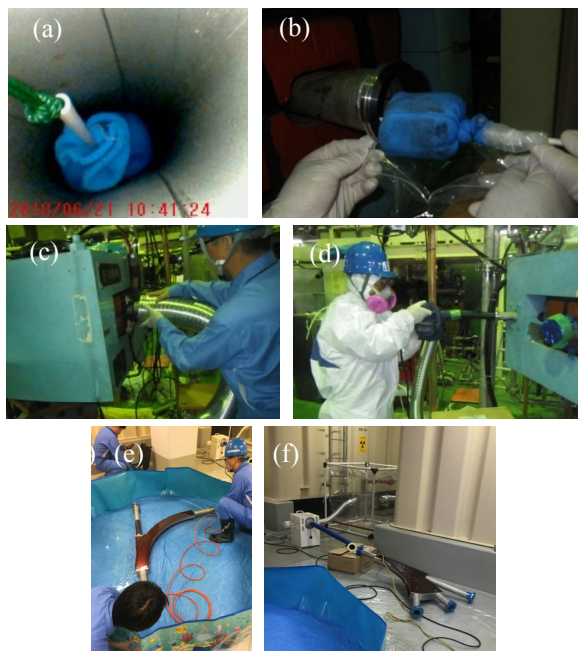
Figure 9: Pictures of cleanings of ducts and chambers in the HEBT; alcohol wiping (a,b), air blowing (c), and vacuuming (d). Two bending magnet chambers were rinsed with pressurized ultra-pure water (e,f).
