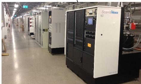
Figure 11: Klystron gallery with K300 modulator.
