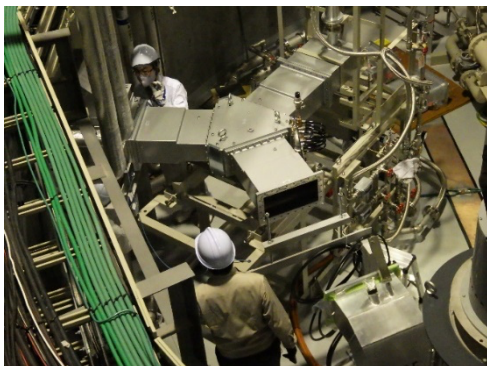
Figure 3: Install of the new 500 MHz RF circulator for storage ring.
